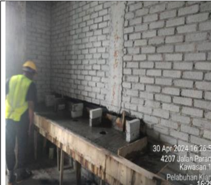
Concrete counter top at female & male toilet 2 nd floor
