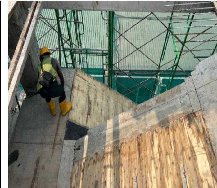
Install formwork for staircase 1 at 5 th floor to 6 th floor
