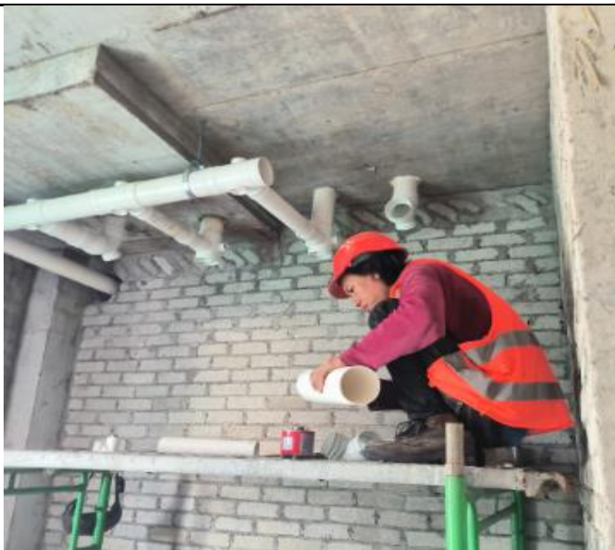
Install sanitary pipe at toilet male 3 rd floor
