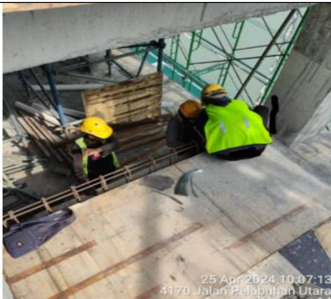
Installing landing beam rebar at staircase 1 5 th floor
