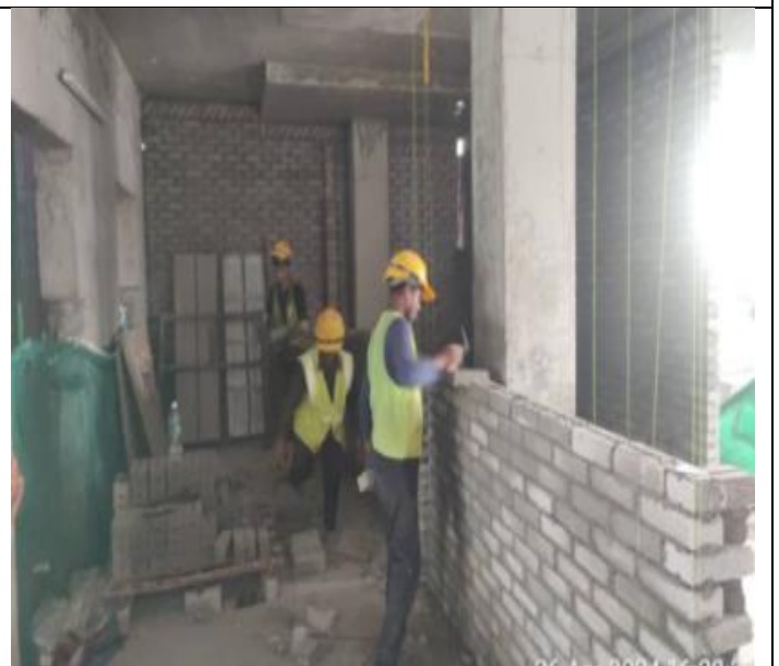
Brickwork at electric riser, data/tel and janitor at 4 th floor
