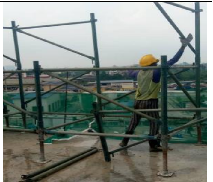
Install c60 shoring at 6 th floor
