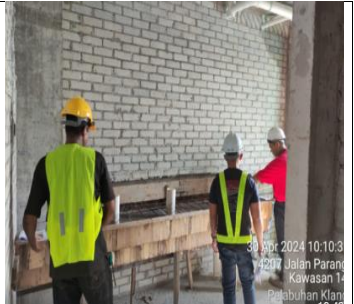
Inspection counter top before concrete at male & female toilet 2 nd floor by En. Zikri
