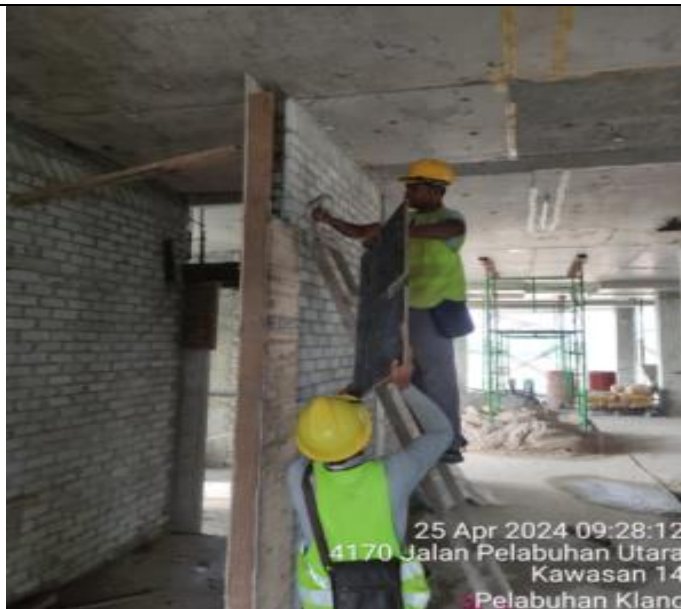
Installing formwork stiffener at female toilet 4 th floor
