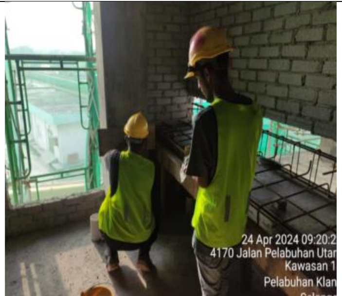
Installing formwork for counter top at female toilet 4 th floor
