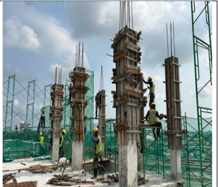
Install formwork for 2 nd lift column at 6 th floor
