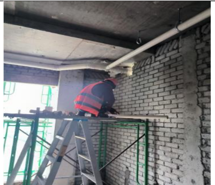
Install sanitary pipe at toilet 3 rd floor
