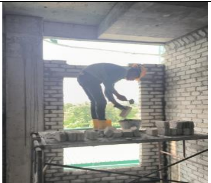
Brickwork at 4 th floor
