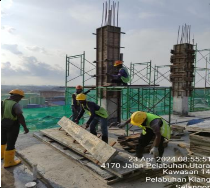
Install formwork for 2 nd lift column at 6 th floor
