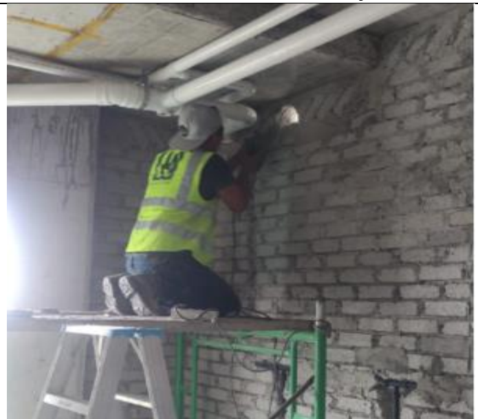
Install sanitary pipe at toilet (female) 4 th floor
