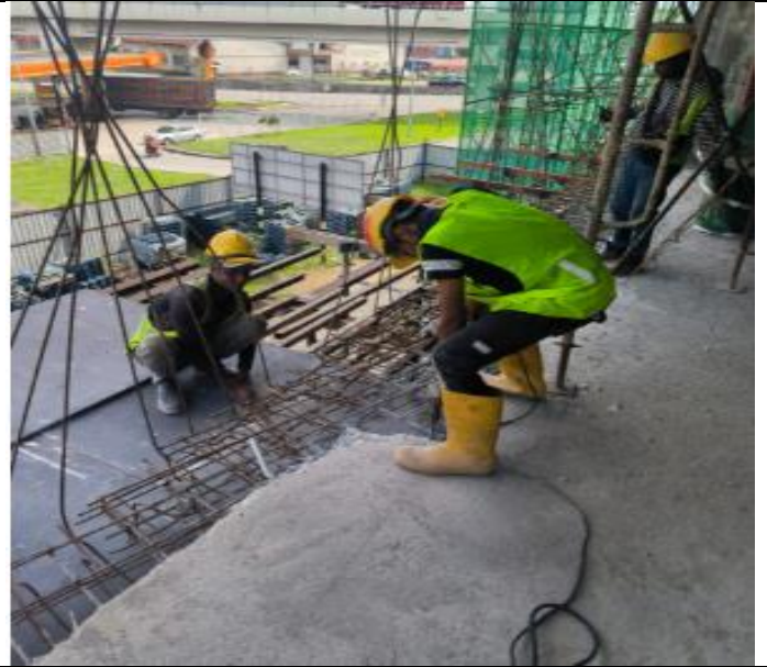
Hacking slab for beam copping at 2 nd floor
