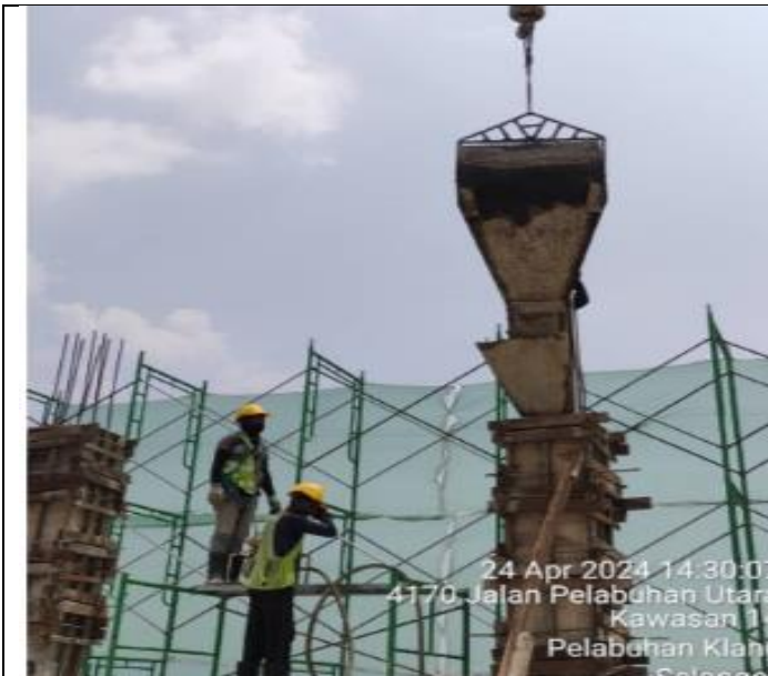
Concrete column at 6 th floor
