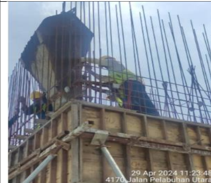
Concrete lift at liftcore 6 th floor
