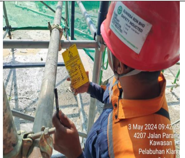
Inspection for perimeter scaffolding by HSO & SSS
