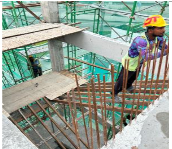
Install formwork for staircase 2 at 5 th floor to 6 th floor
