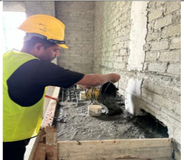
Concreting counter top at female toilet 1 st floor
