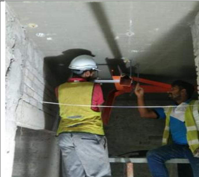
Install trunking at ground floor
