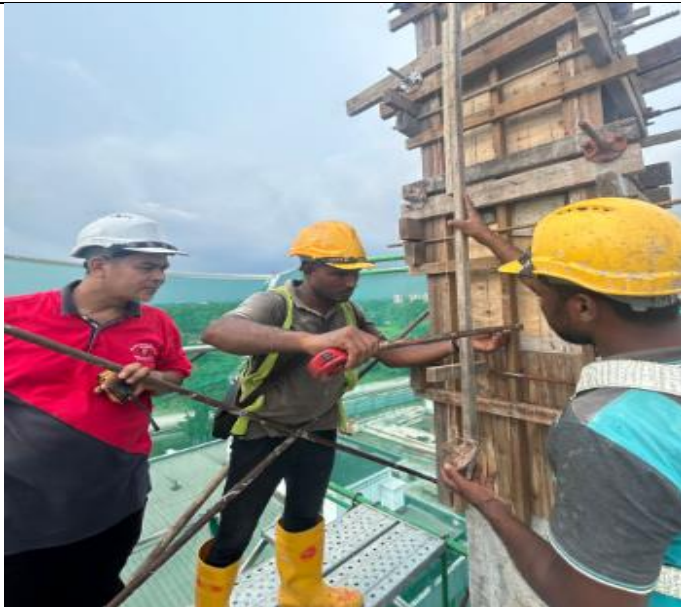
Inspection column vertically at 6 th floor by En. Zikri
