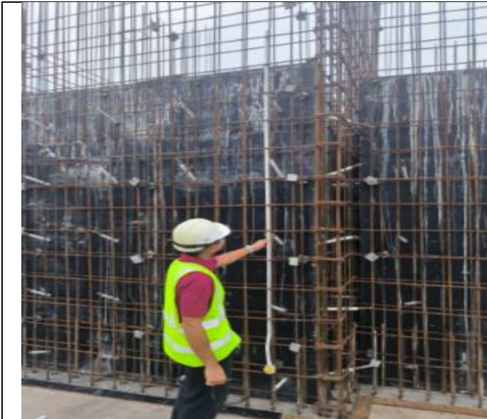
Inspection conduit at liftcore at 6 th floor by En. Muz
