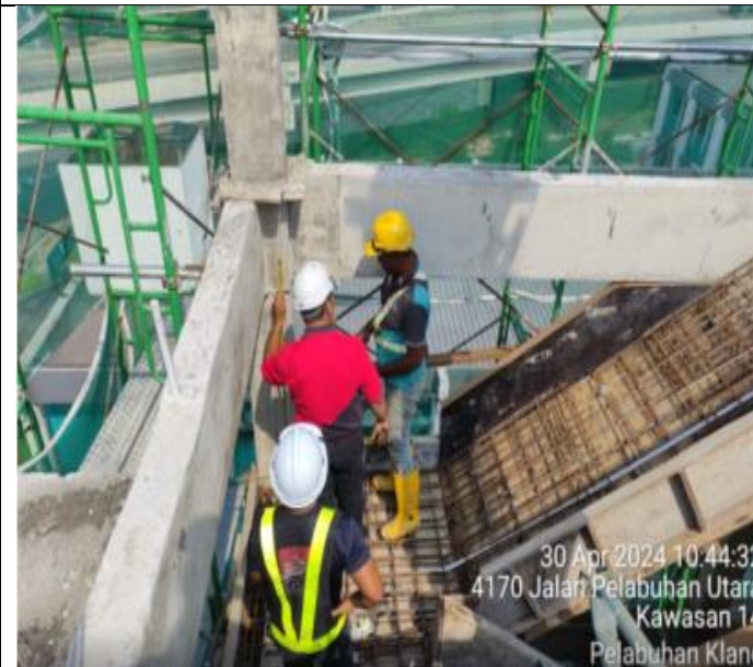
Inspection formwork staircase 1&2 at 5 th floor to 6 th floor by En. Zikri
