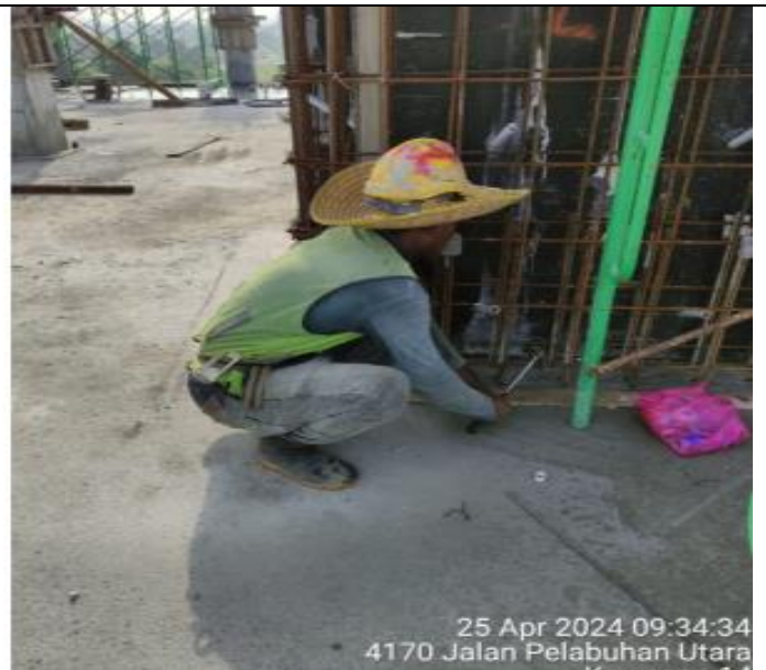
Install base lift formwork at liftcore 6 th floor
