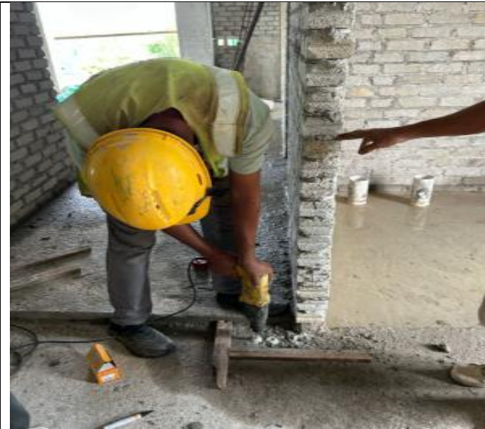
Install stiffener rebar at female toilet 4 th floor
