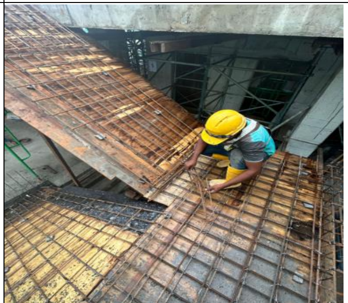
Install rebar for staircase 1 at 5 th floor to 6 th floor
