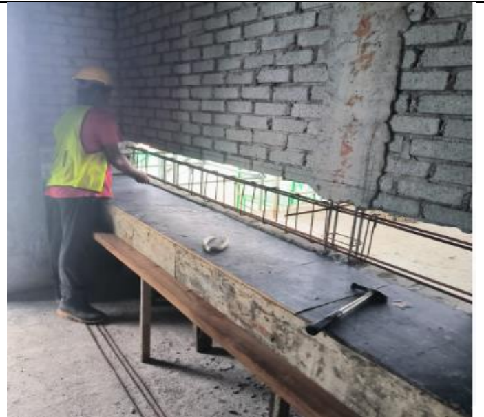
Install rebar for counter top at toilet female 2 nd floor
